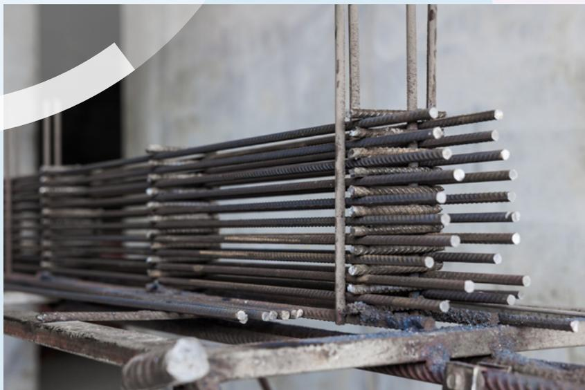
CES TREILLIS OU CAGES AINSI ASSEMBLÉS SERONT DISPOSÉS DANS UN COFFRAGE DANS LEQUEL SERA COULÉ LE BÉTON. LA PROFESSION DES **ARMATURIERS** S'EST SPÉCIALISÉE DANS LA RÉALISATION DE CES ARMATURES MÉTALLIQUES.
